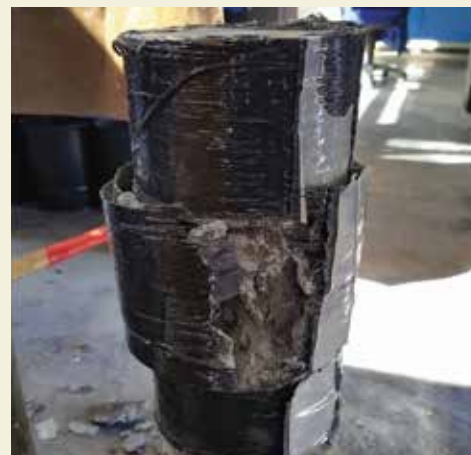
Figure 1: CFRP reinforced cylinder concrete sample, after compression test
