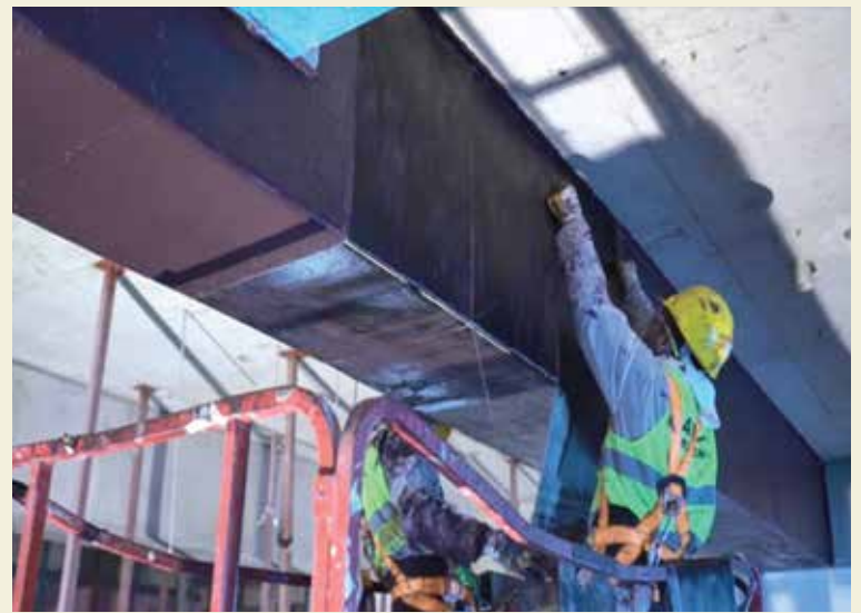
Figure 7: A full-scale application, reinforcing of a concrete beam
